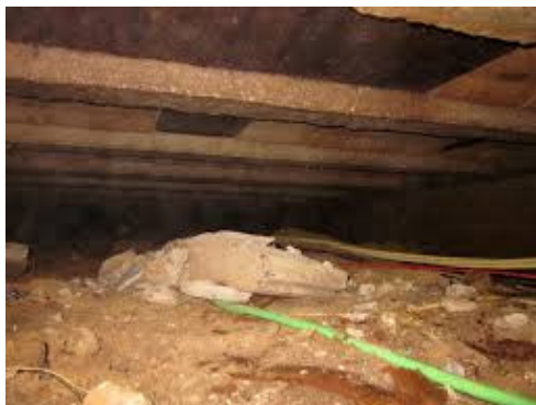
Figure 2: Typical crawlspace. Source Woonbron
