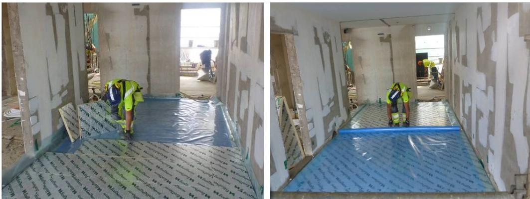
Figure 4 Assembly of PIR insulation as floating floor structure. Mounting of first layer on plastic foil (left) and covering second layer with another sheet of plastic foil (right).
