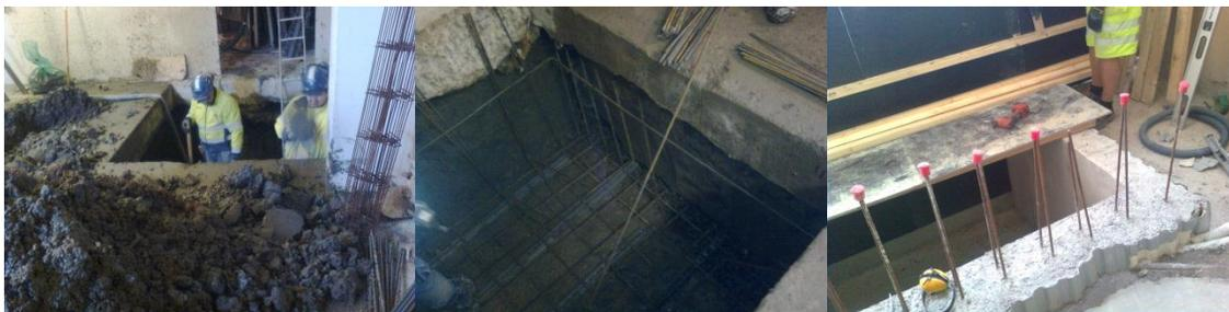
Figure 5 Some of the operations involved for elevator pits. Left: Excavating by hand inside a building. Center: Reinforcement on the gravel floor. Right: After excavation and casting of pit, House J
