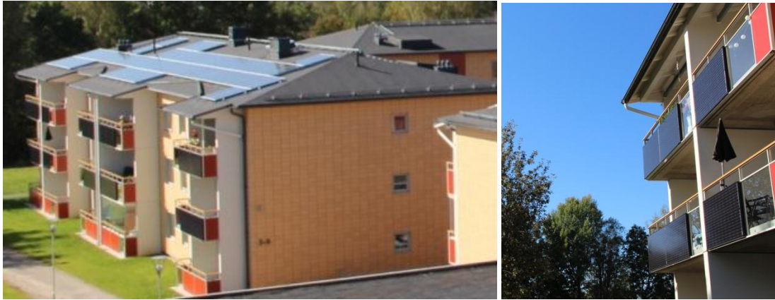
Figure 4 PV cells mounted on roof tops and balcony fencing.
