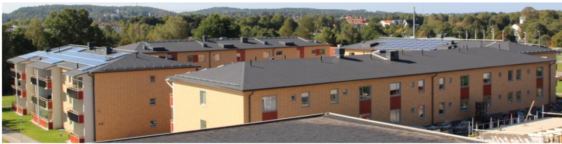
Figure 3 Final skyline of Alingsås rooftops for Houses N,Q,O,P. The PV cells of houses N and P, facing east, is very visible from a bird's view but not from the ground. The elevator rooftops of houses Q and N are identified by the shadows from this perspective, but neither of them are very clearly seen from the ground.
